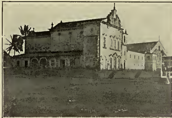
CHAPEL OF NOSSA SENHORA DA GRAÇA, BAHIA, BUILT BY PARAGUASSÚ.
