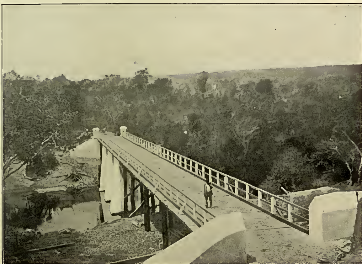
BRIDGE CROSSING RIO UNA, STATE OF BAHIA.
