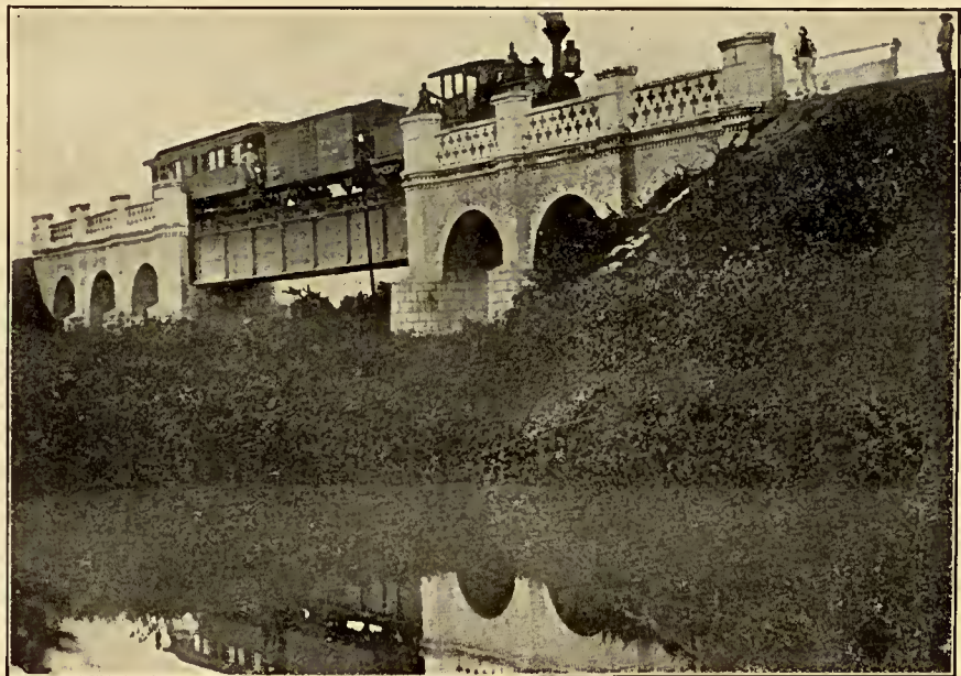
RAILROAD BRIDGE OF ACARAHÚ, CEARÁ.
