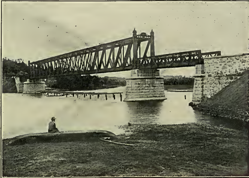
RAILWAY BRIDGE AT CASTRO, STATE OF PARANA.
