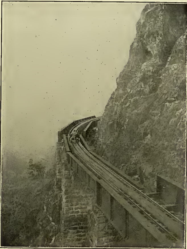
VIADUCT ON THE PARANA RAILWAY.
